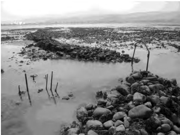
Figure 18 Large stone fish weir at Minehead Bay, Somerset, with a 'hoop' of welded scaffolding poles above the gut or outflow channel. Note too the iron poles outside the apex.
