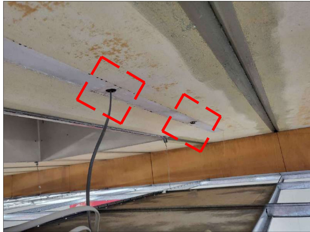
PHOTO 62 - PLANK No. 160 2No. SERVICE HOLES
