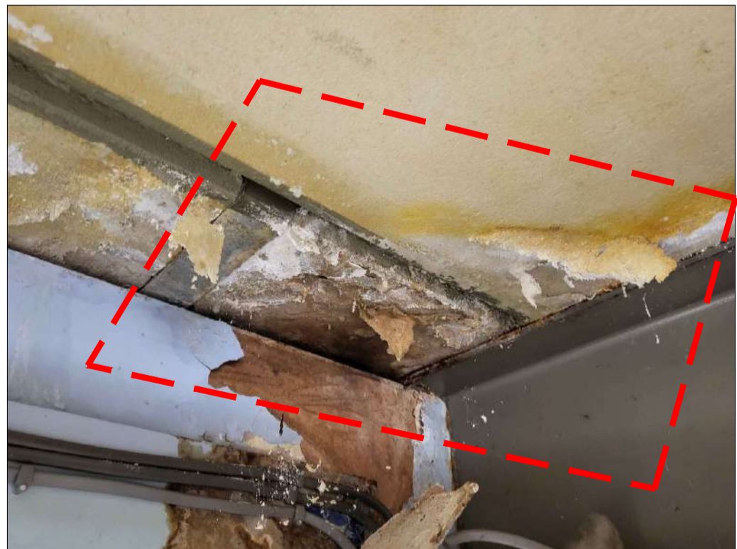
PHOTO 28 - PLANK No. 58 DELAMINATION/EFFLORESCENCE AT END 2 BRACKET AT END 2
