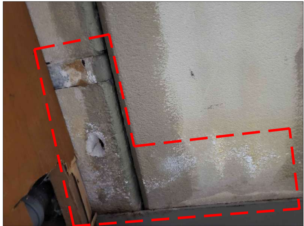
PHOTO 83 - PLANK No. 209 & 175 BRACKET HOLE AT END 1 EFFLORESCE AT BOTH ENDS
