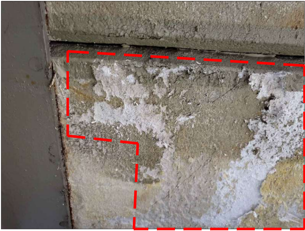
PHOTO 2 - PLANK No. 1 DELAMINATION/EFFLORESCENCE AT ENDS 1 & 2
