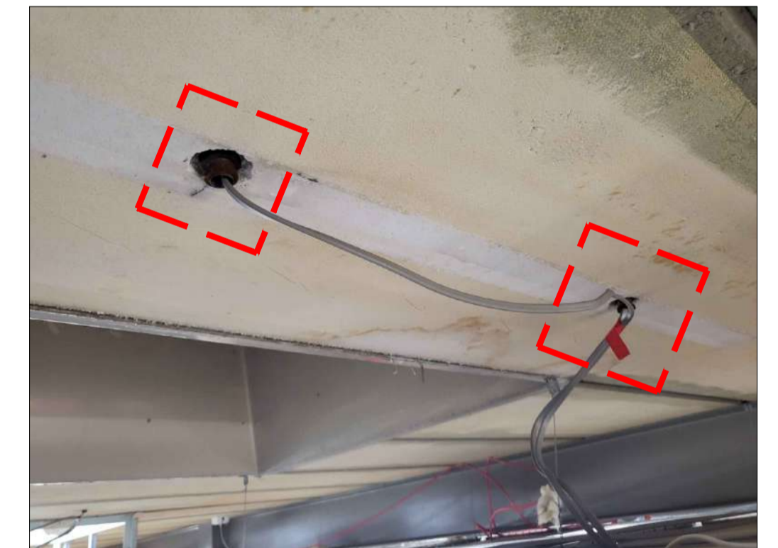
PHOTO 55 - PLANK No. 130 2No. SERVICE HOLES
