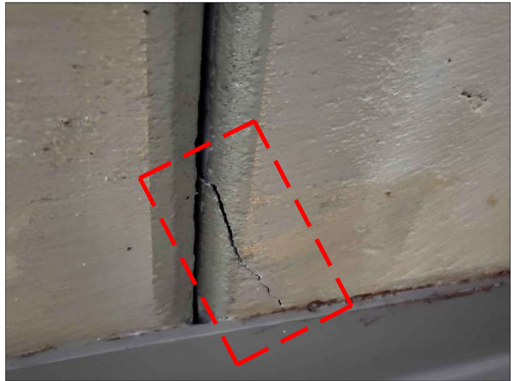
PHOTO 82 - PLANK No. 204 CRACK AT END 2
