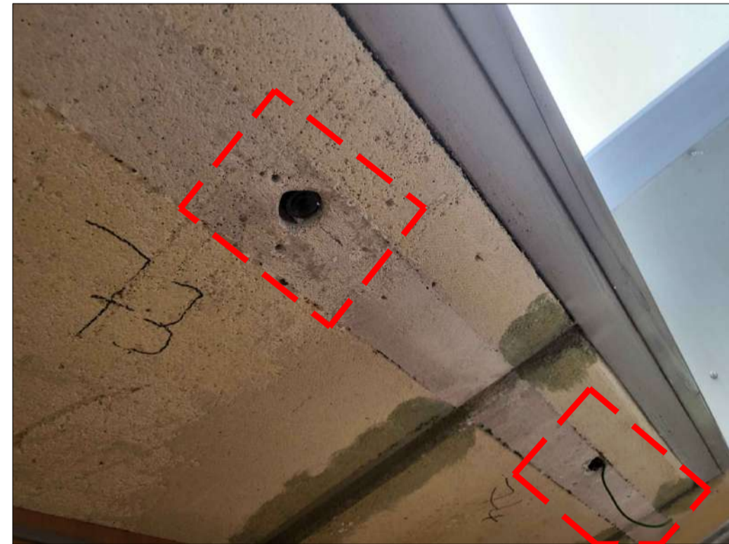
PHOTO 36 - PLANK No. 73 & 74 SERVICE HOLES
