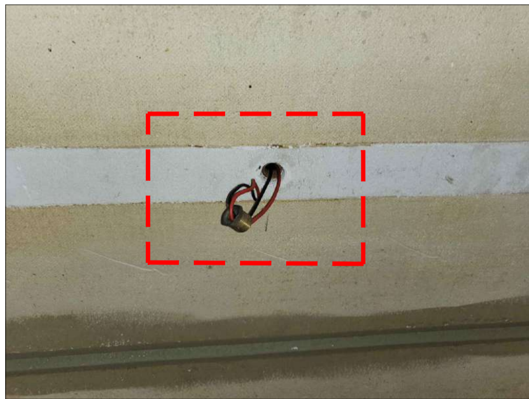
PHOTO 96 - PLANK No. 213 1No. SERVICE HOLE
