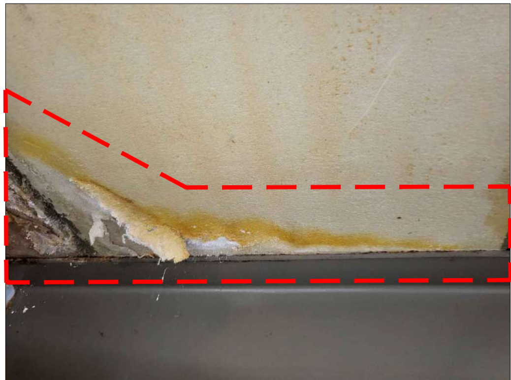
PHOTO 27 - PLANK No. 57 DELAMINATION/EFFLORESCENCE AT END 2
