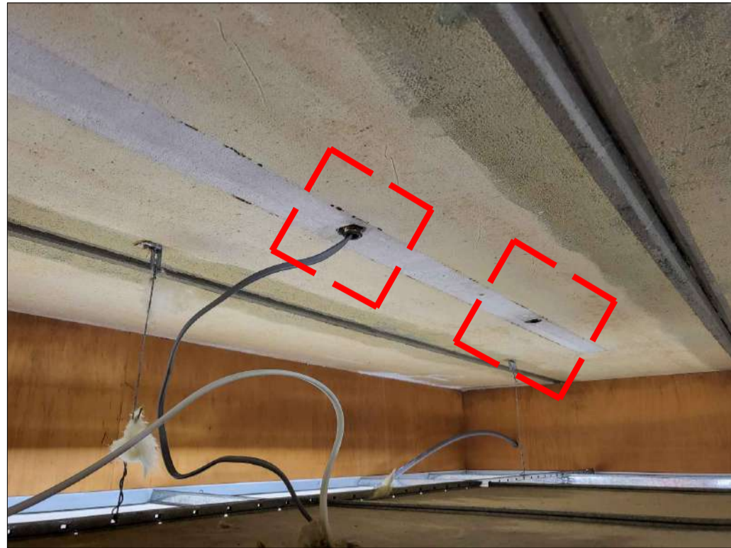
PHOTO 63 - PLANK No. 164 2No. SERVICE HOLES
