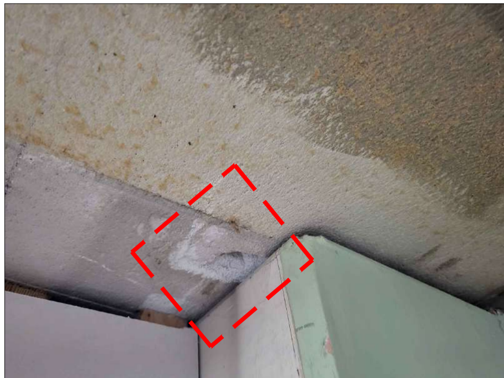
PHOTO 75 - PLANK No. 191 HOLE AT END 1
