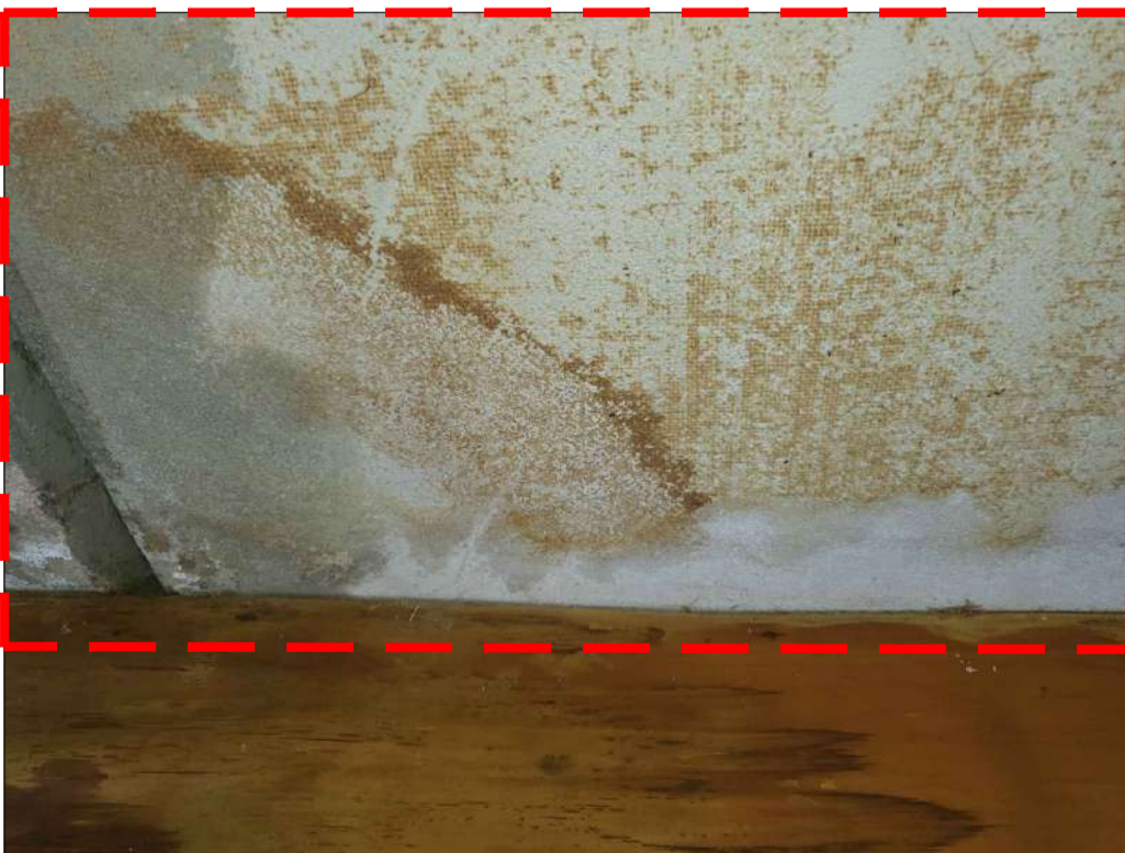
PHOTO 103 - PLANK No. 232 WATER STAIN AT END 2 BY OLD COLLAPSED CEILING TILE
