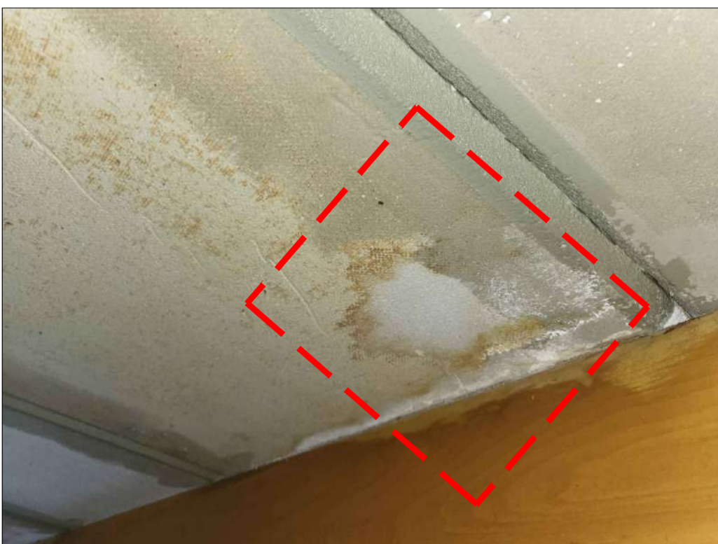
PHOTO 105 - PLANK No. 234 WATER STAIN AT END 2
