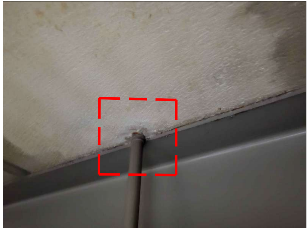
PHOTO 78 - PLANK No. 198 HOLE AT BEARING END 2
