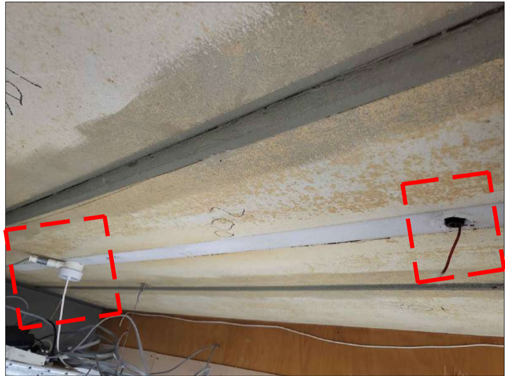
PHOTO 77 - PLANK No. 200 2No. SERVICE HOLES
