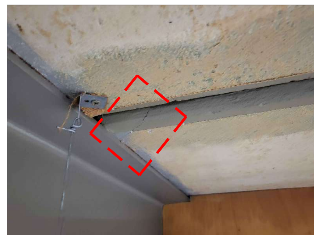
PHOTO 58 - PLANK No. 139 CRACK AT END 1
