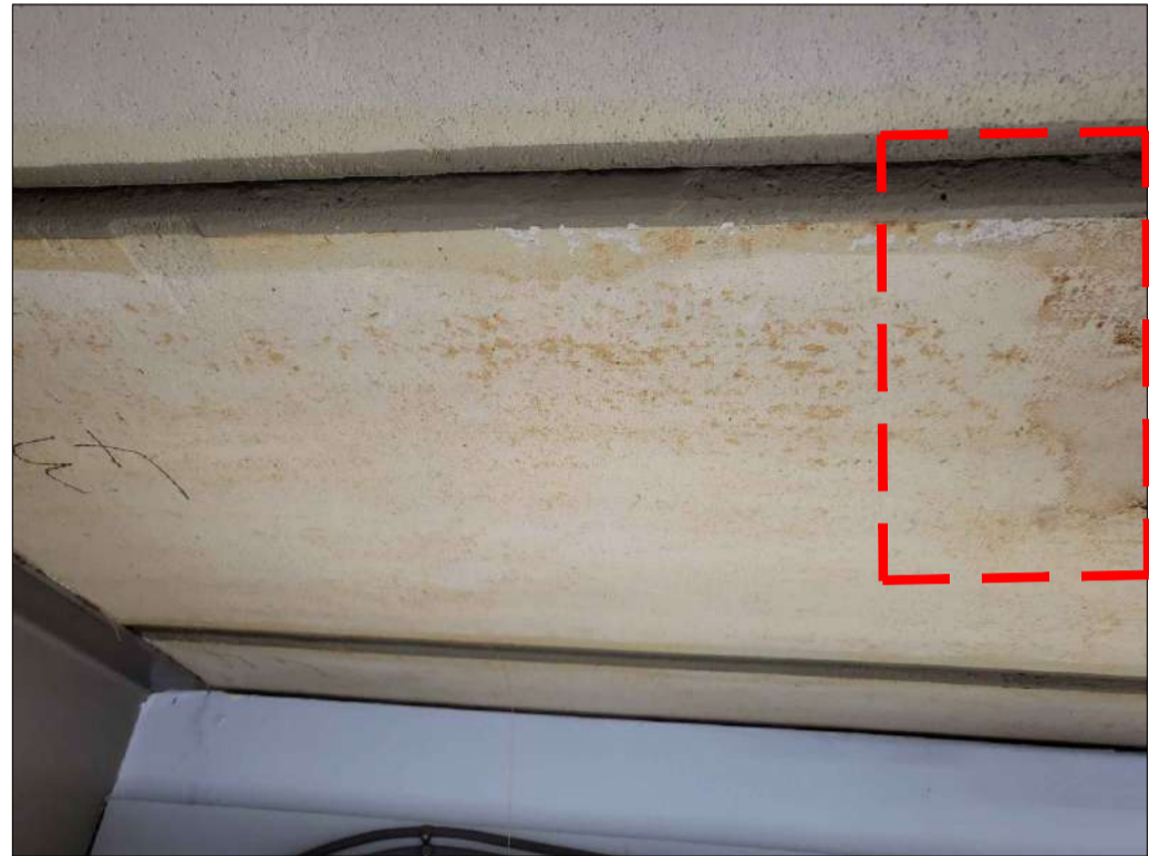
PHOTO 17 - PLANK No. 43 POSSIBLE WATER STAINS AT END 1
