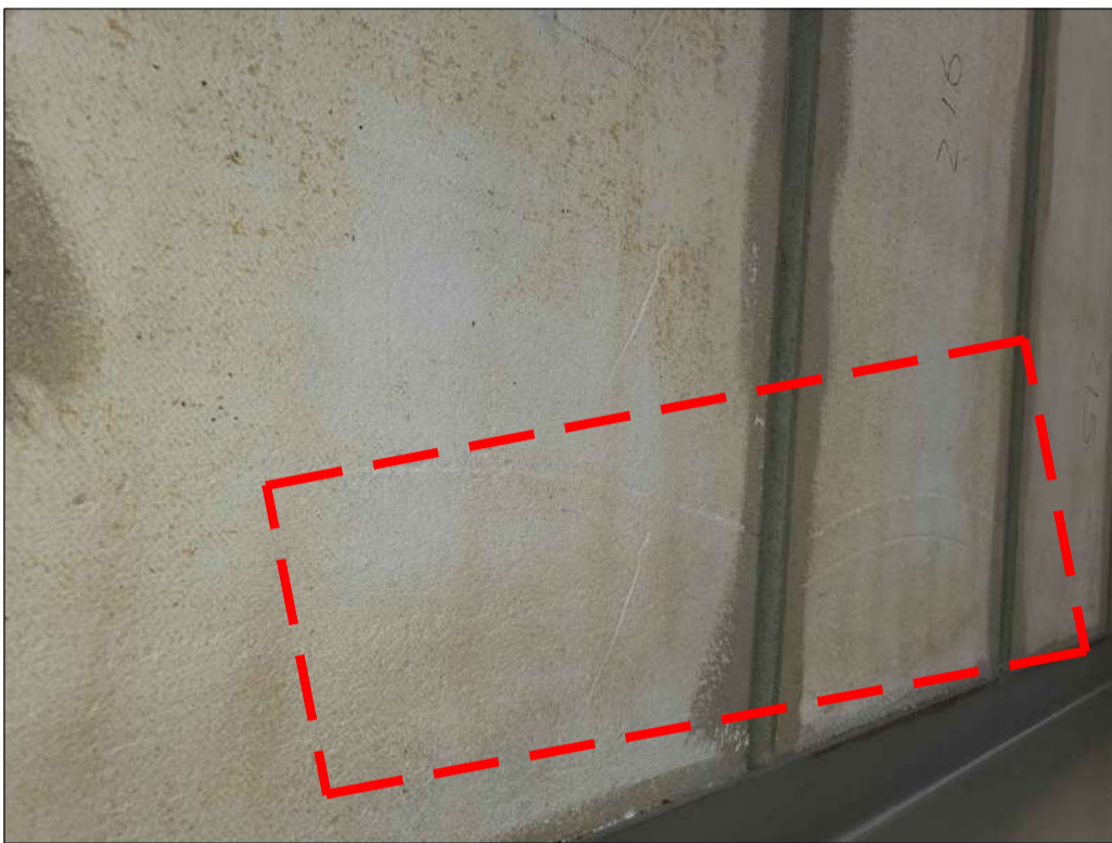
PHOTO 93 - PLANK No. 216 & 217 SCAR AT END 1
