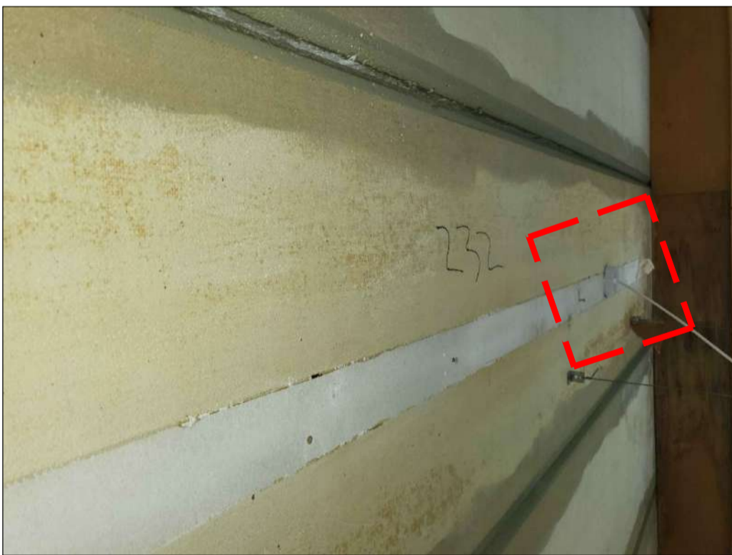
PHOTO 98 - PLANK No. 232 1No. HOLE
