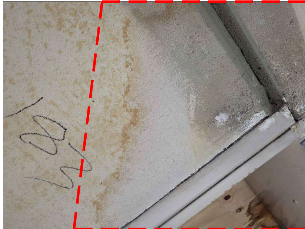
PHOTO 69 - PLANK No. 183 DELAMINATION WATER STAIN
