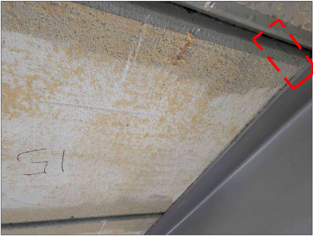
PHOTO 4 - PLANK No. 15 CRACK AT END 2
