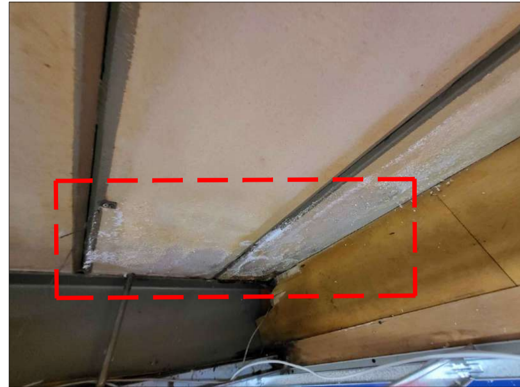
PHOTO 31 - PLANK No. 47 & 48 RUST STAIN EFFLORESCENCE AT END 2
