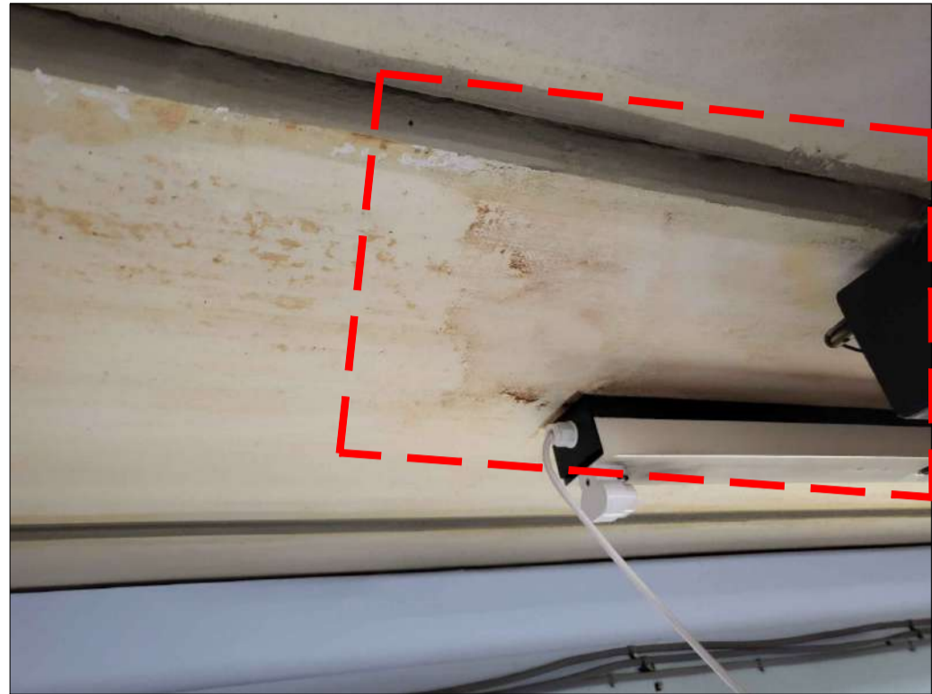
PHOTO 16 - PLANK No. 43 POSSIBLE WATER STAINS AT END 1
