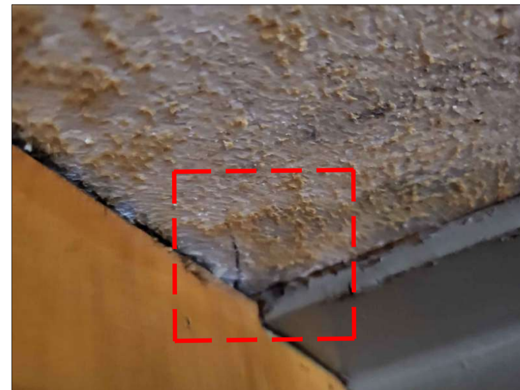
PHOTO 53 - PLANK No. 122 CRACK AT END 1
