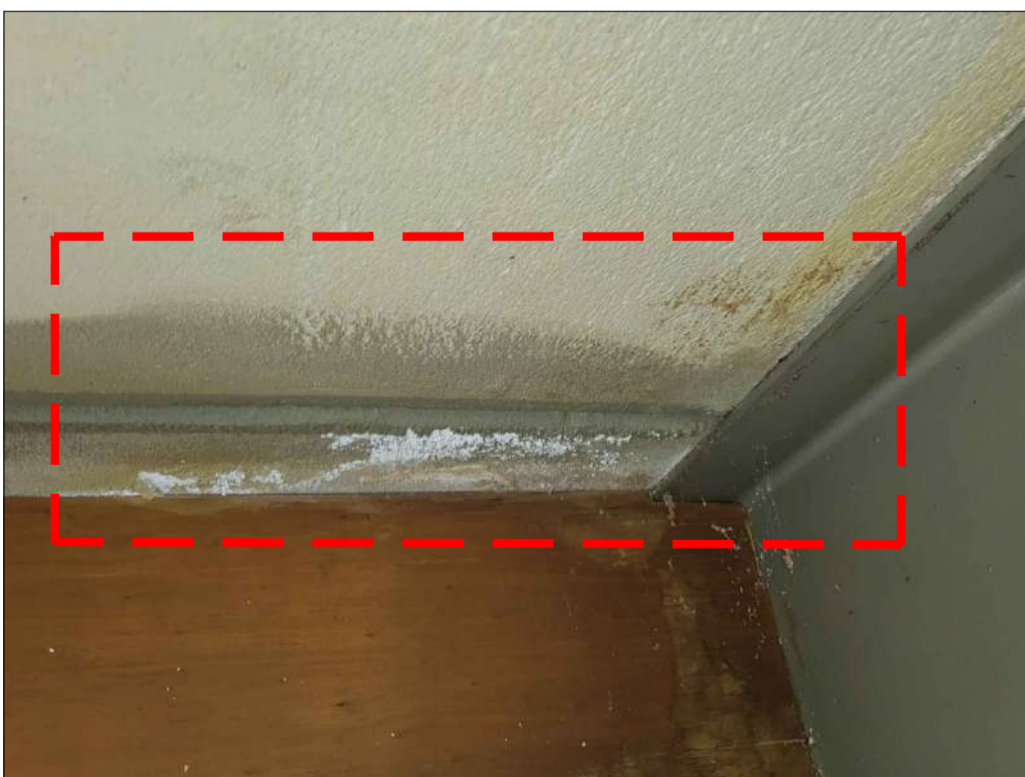
PHOTO 102 - PLANK No. 238 DELAMINATION/EFFLORESCENCE AT END 1
