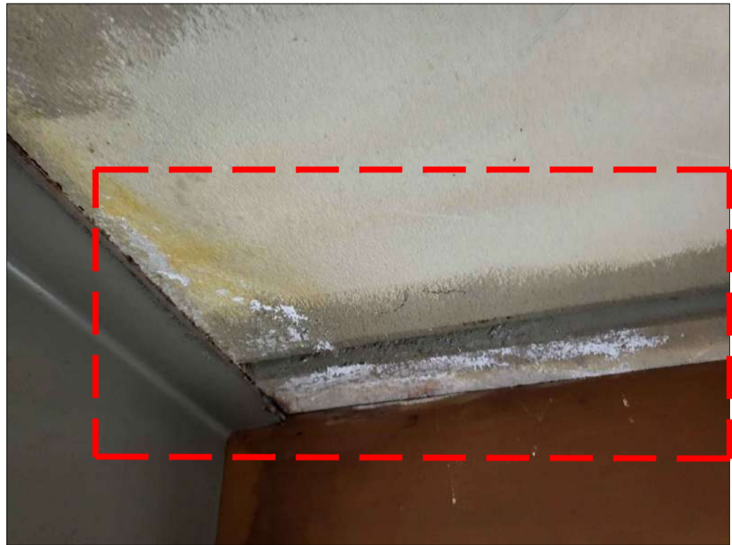
PHOTO 85 - PLANK No. 175 & 209 EFFLORESCE AT BOTH ENDS
