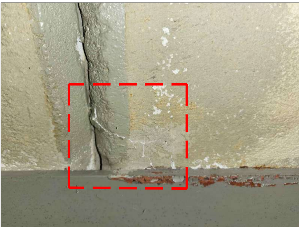
PHOTO 100 - PLANK No. 236 CRACK AT END 1
