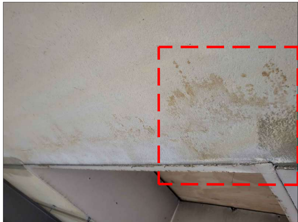
PHOTO 86 - PLANK No. 207 WATER STAIN
