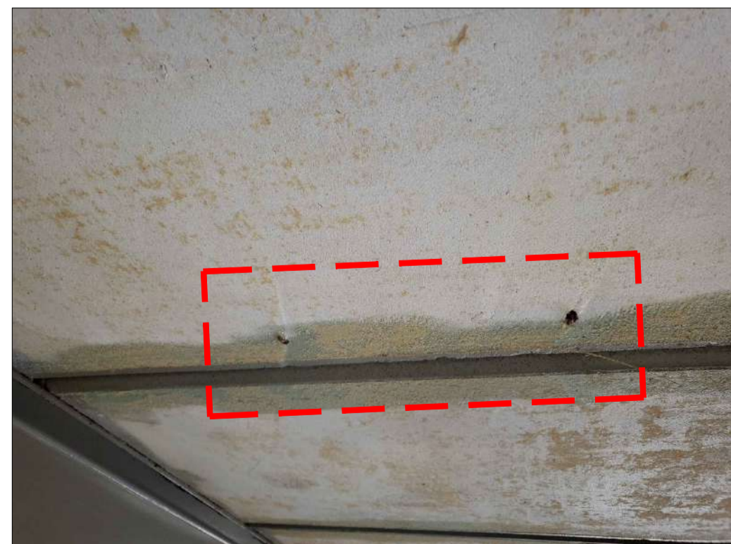
PHOTO 42 - PLANK No. 90 EXPOSED STEEL AT IRREGULAR CENTRES
