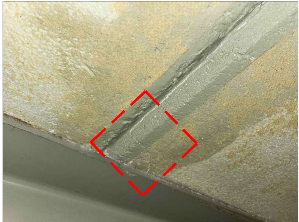
PHOTO 80 - PLANK No. 201 CRACK AT END 2
