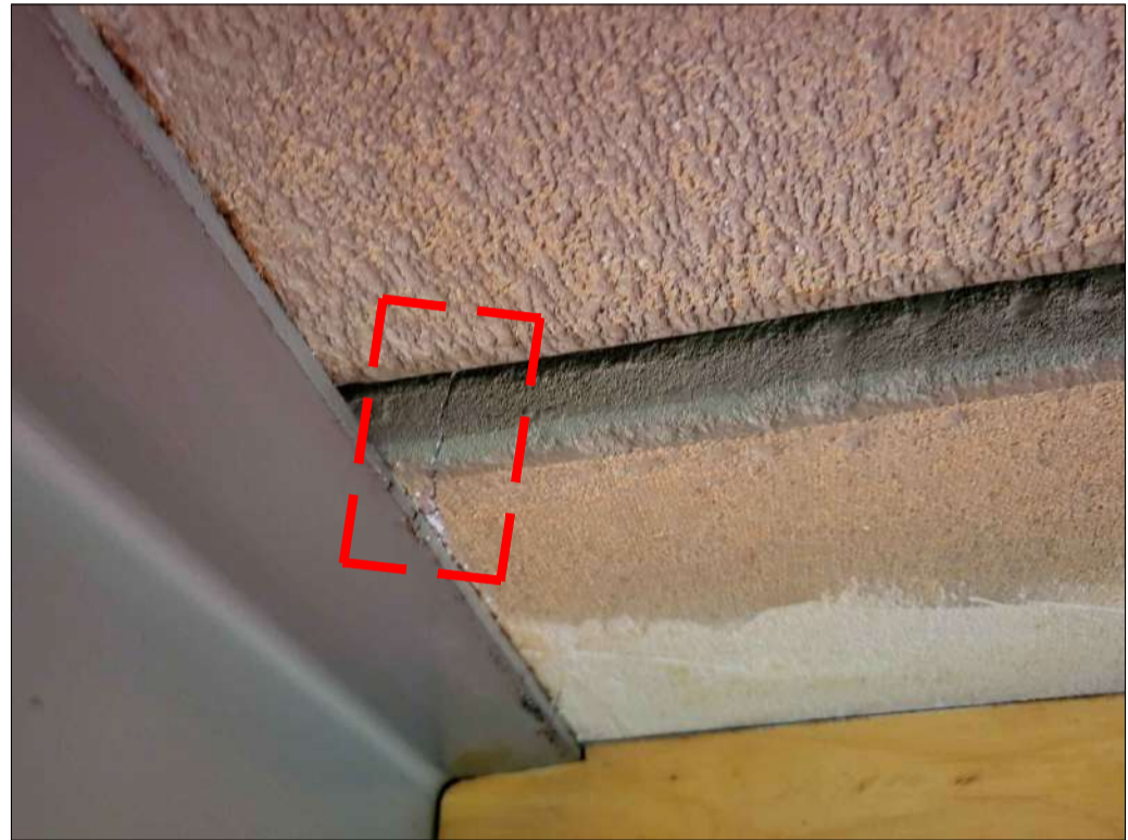
PHOTO 19 - PLANK No. 33 CRACK AT END 2
