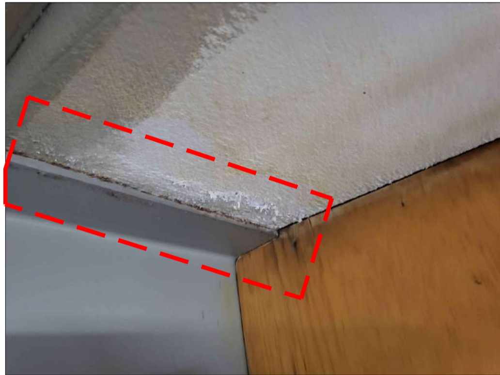
PHOTO 67 - PLANK No. 174 EFFLORESCENCE AT END 1
