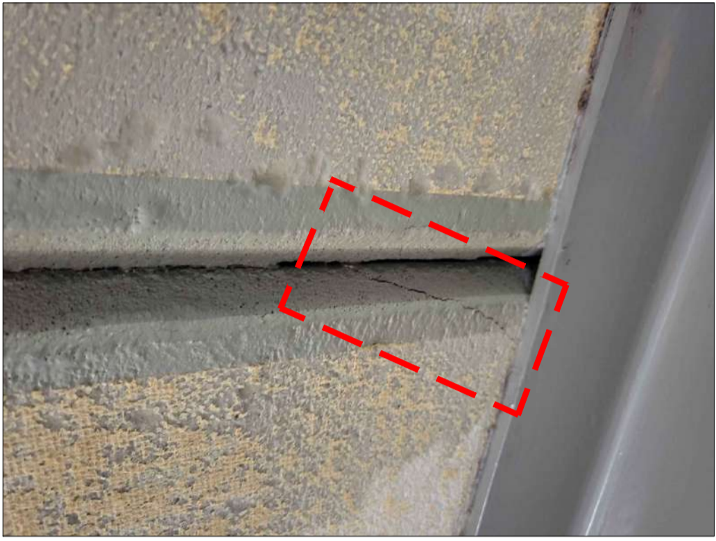
PHOTO 3 - PLANK No. 15 CRACK AT END 2
