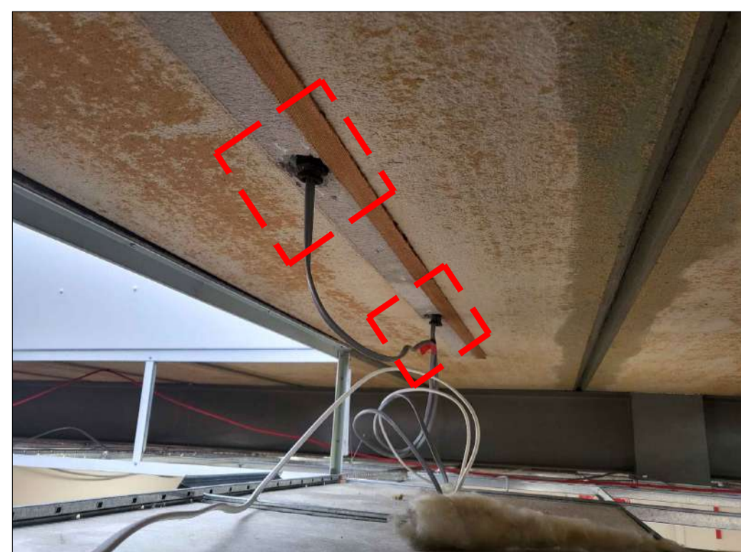
PHOTO 57 - PLANK No. 138 2No. SERVICE HOLES
