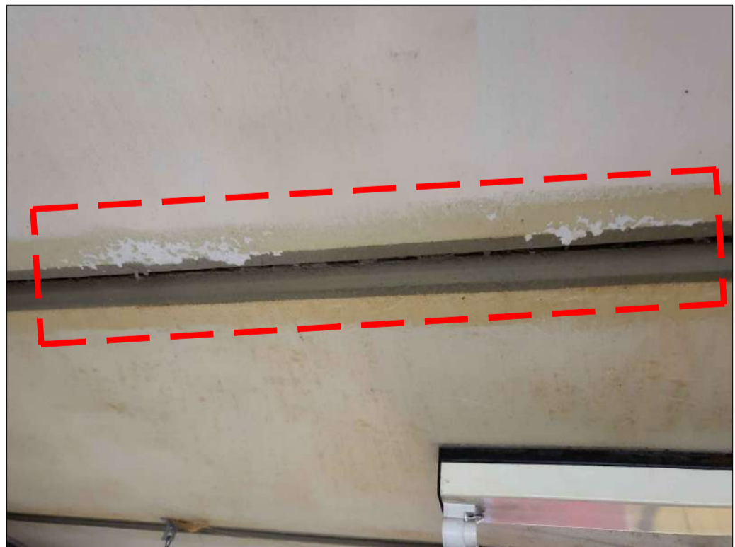
PHOTO 30 - PLANK No. 54 SIDE DELAMINATION/EFFLORESCENCE AT END 2
