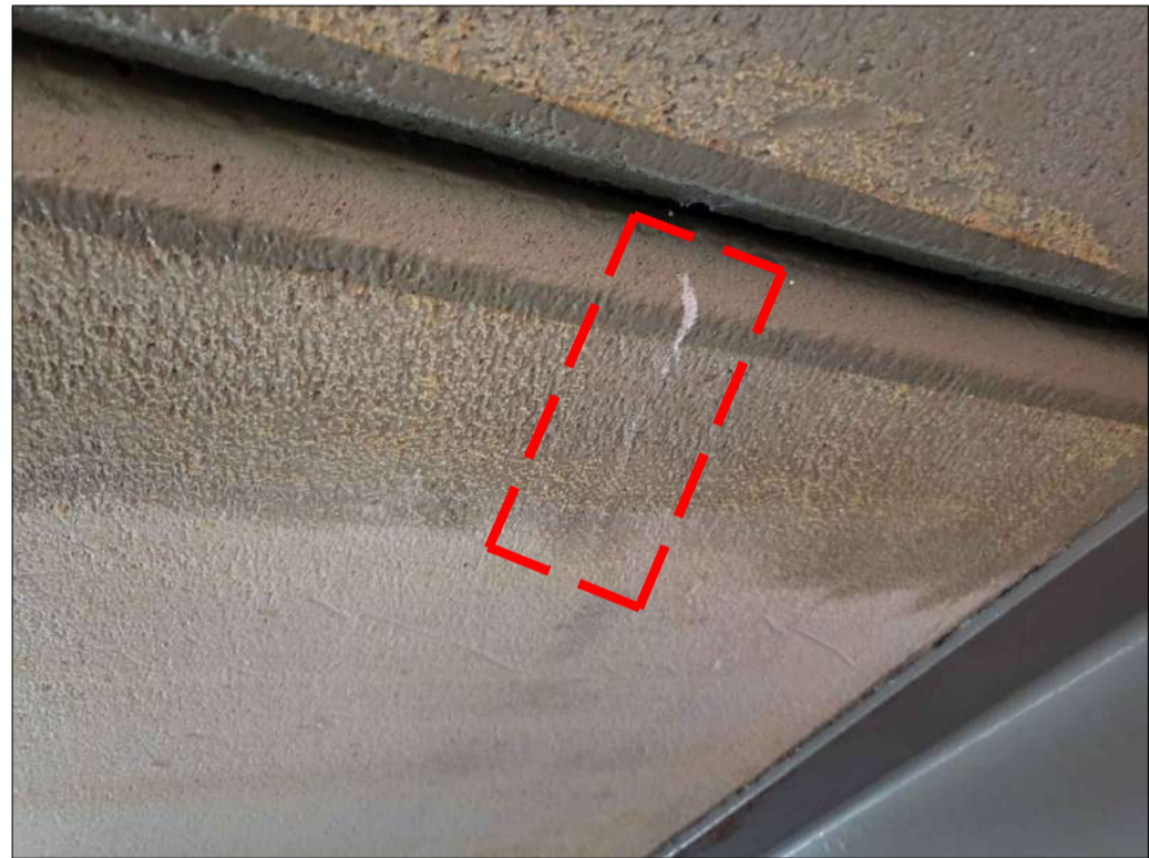
PHOTO 21 - PLANK No. 38 CRACK AT END 2
