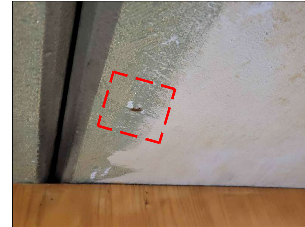
PHOTO 49 - PLANK No. 109 EXPOSED FIXING
