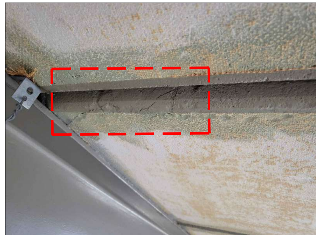
PHOTO 52 - PLANK No. 100 2No. HOLES CRACK AT ENDS 1 & 2
