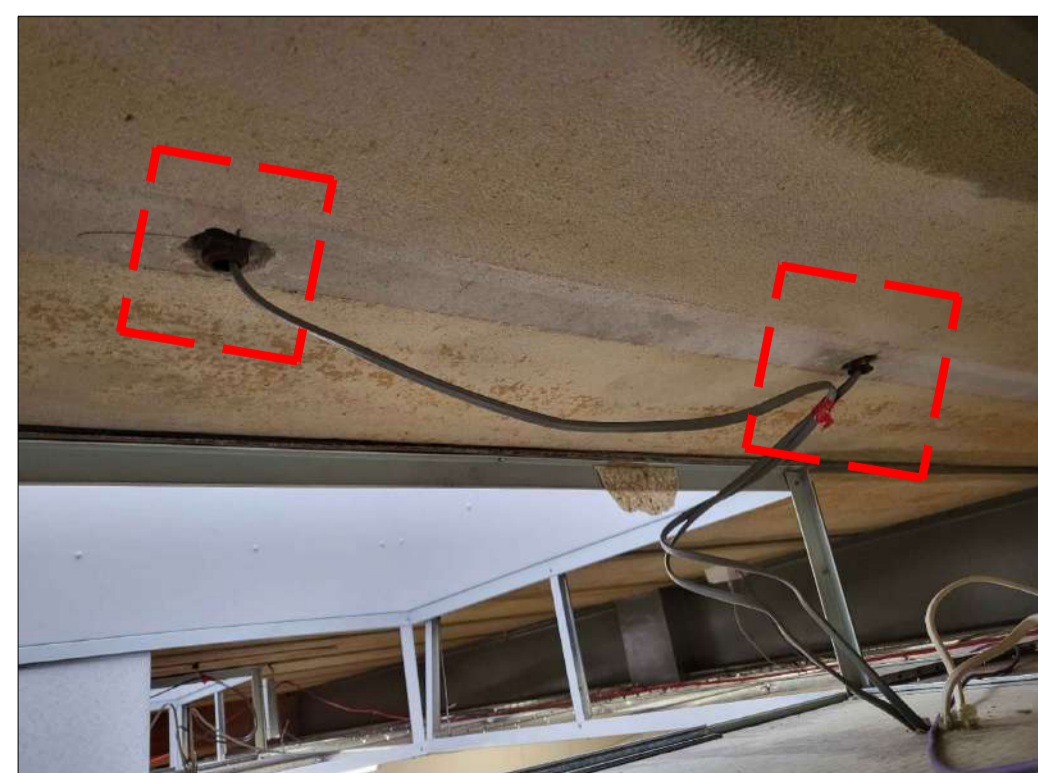
PHOTO 56 - PLANK No. 134 2No. SERVICE HOLES
