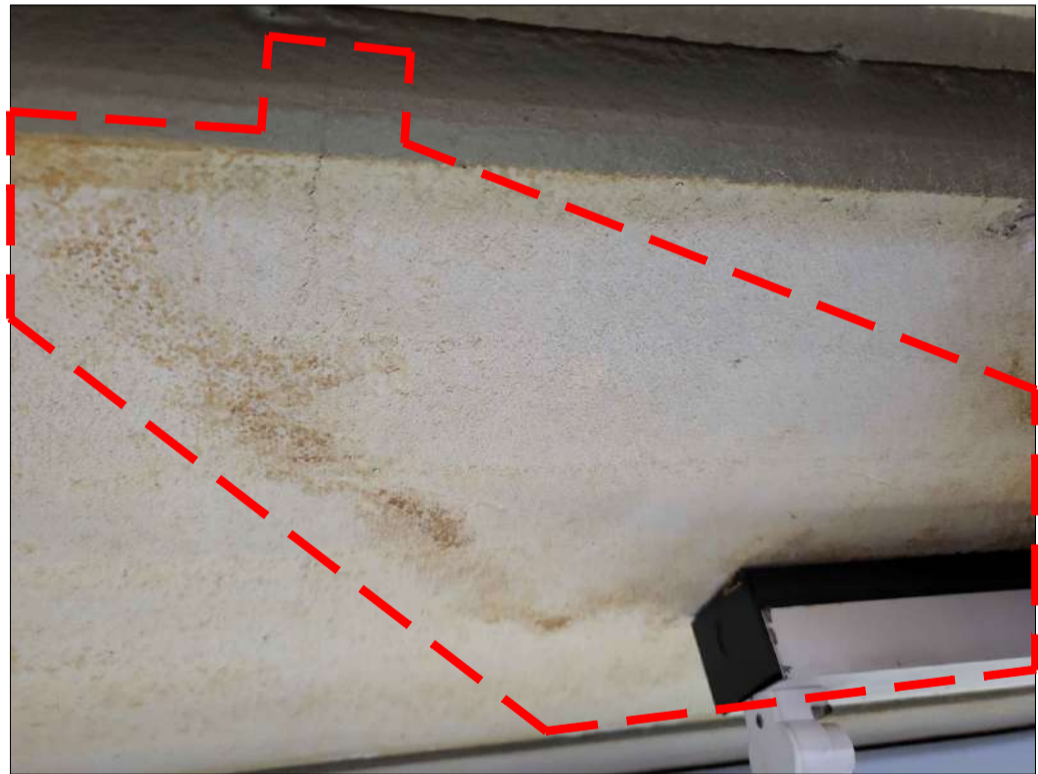
PHOTO 24 - PLANK No. 57 DAMP BY LIGHT CRACK AT END 1
