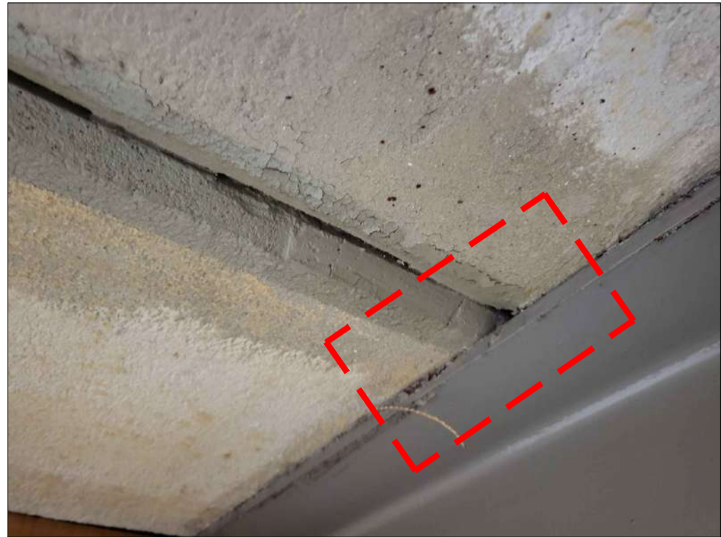
PHOTO 76 - PLANK No. 174 CRACK AT END 2
