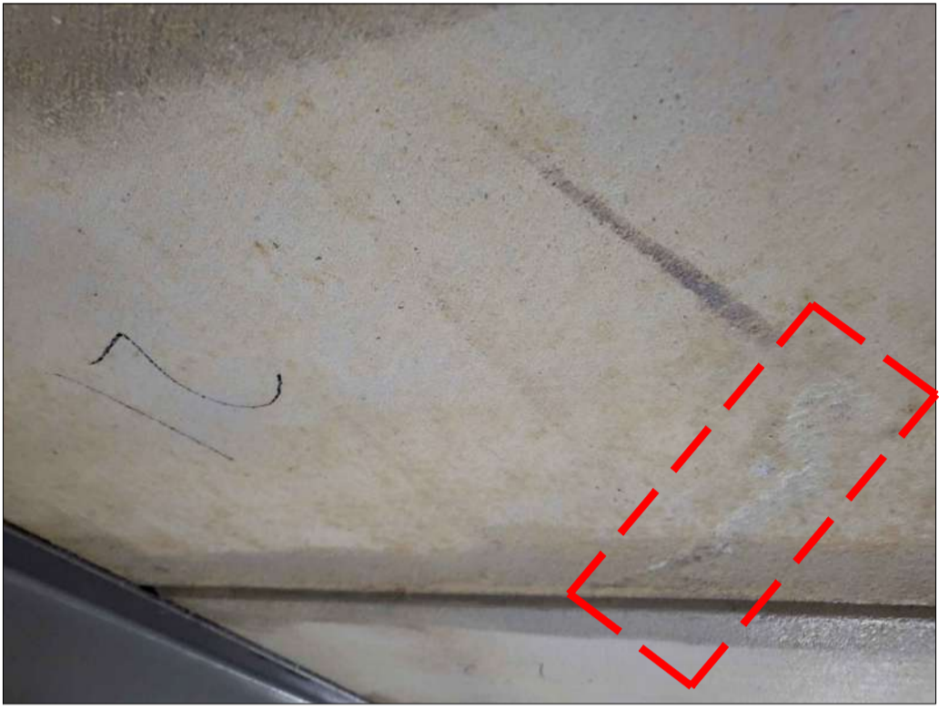
PHOTO 5 - PLANK No. 21 SCARRING AT END 1
