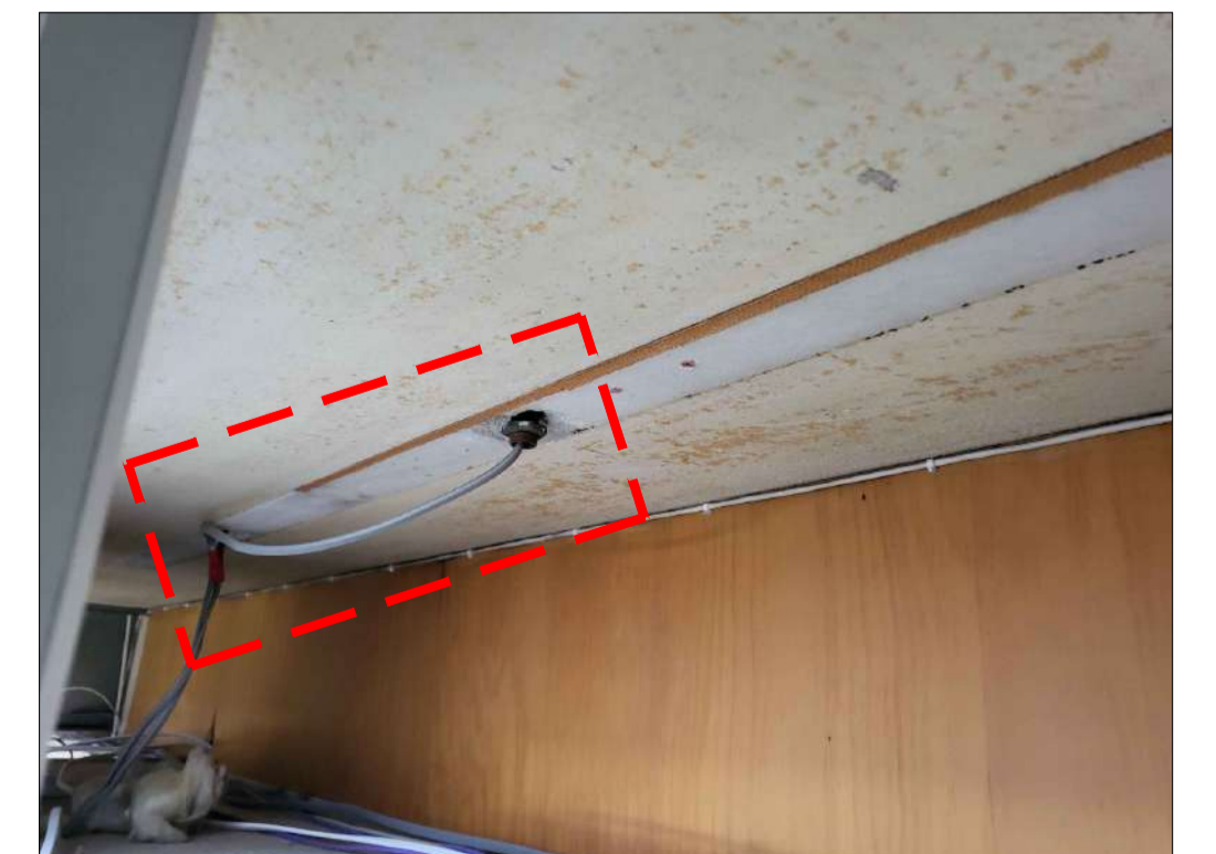
PHOTO 45 - PLANK No. 96 2No. SERVICE HOLES
