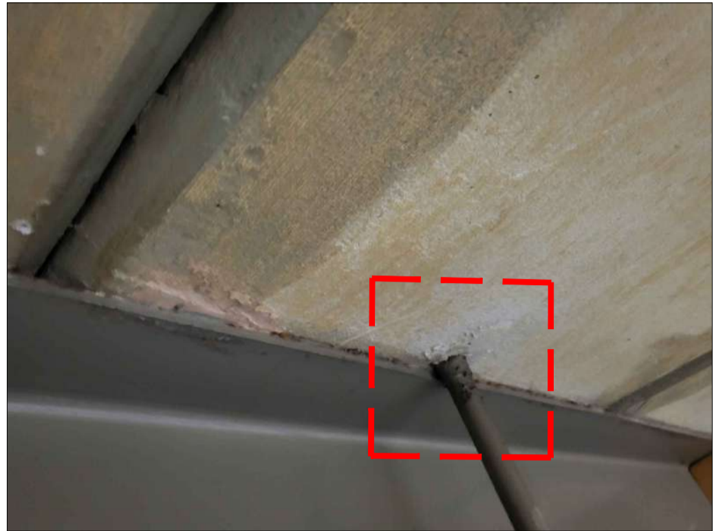
PHOTO 79 - PLANK No. 200 HOLE AT BEARING END 2
