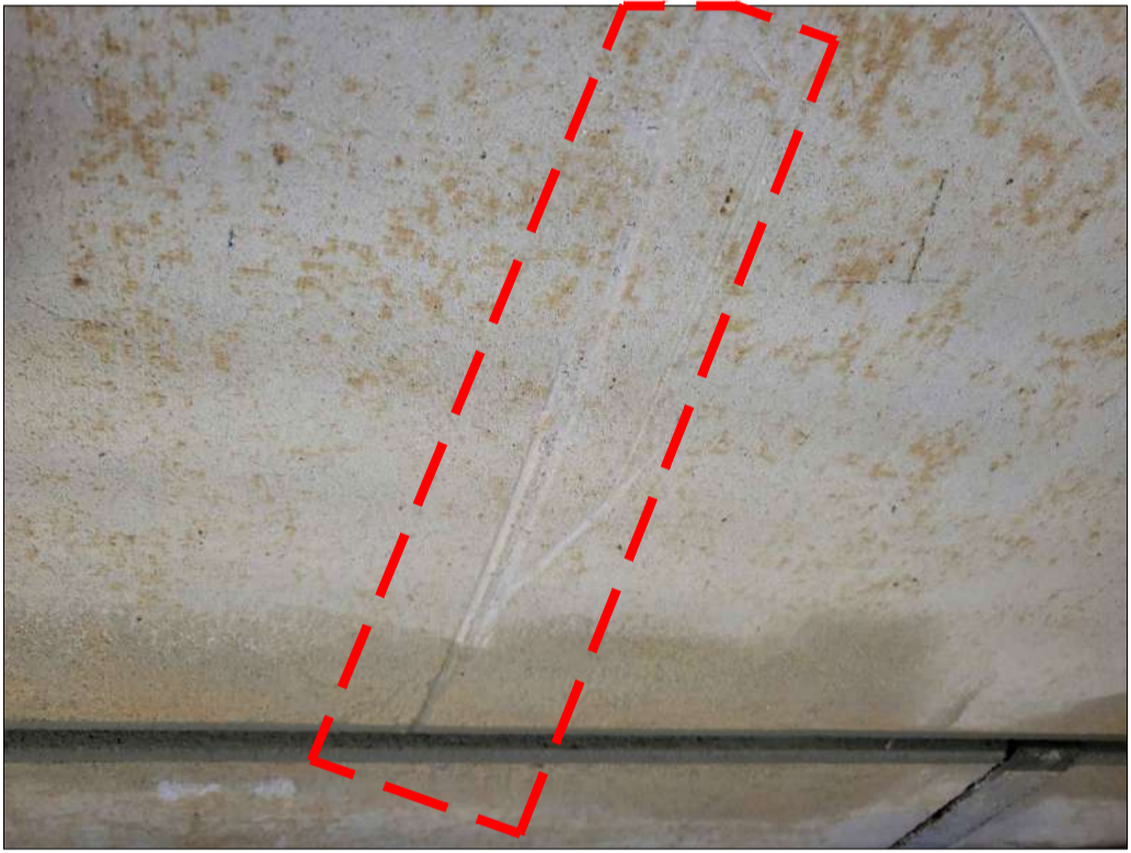
PHOTO 10 - PLANK No. 27 SCARRING AT END 2
