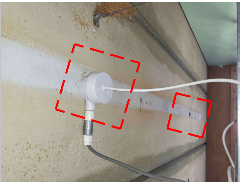
PHOTO 95 - PLANK No. 226 2No. SERVICE HOLES
