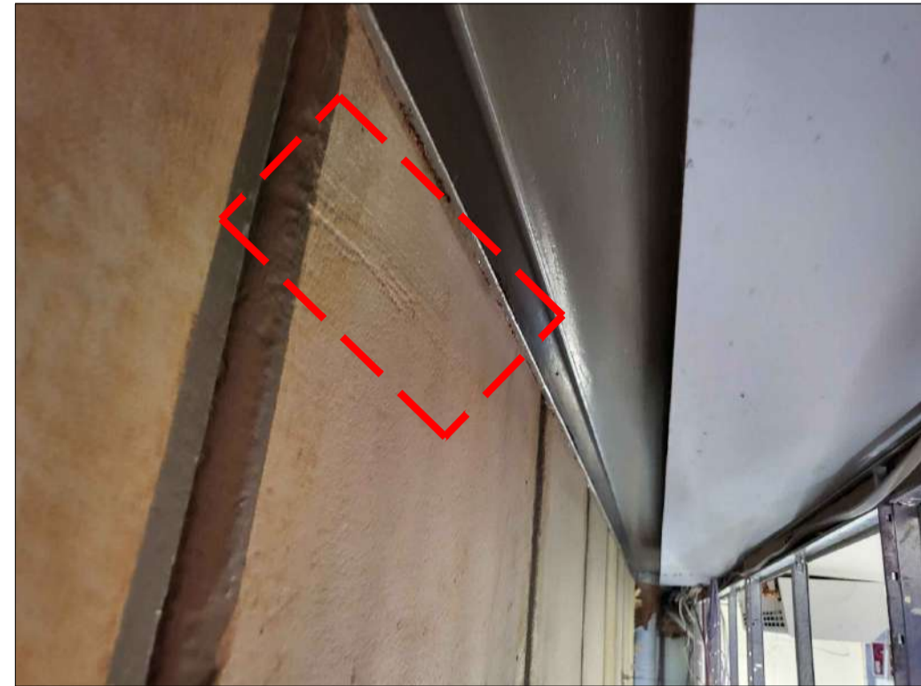
PHOTO 32 - PLANK No. 50 SCARRING AT END 2
