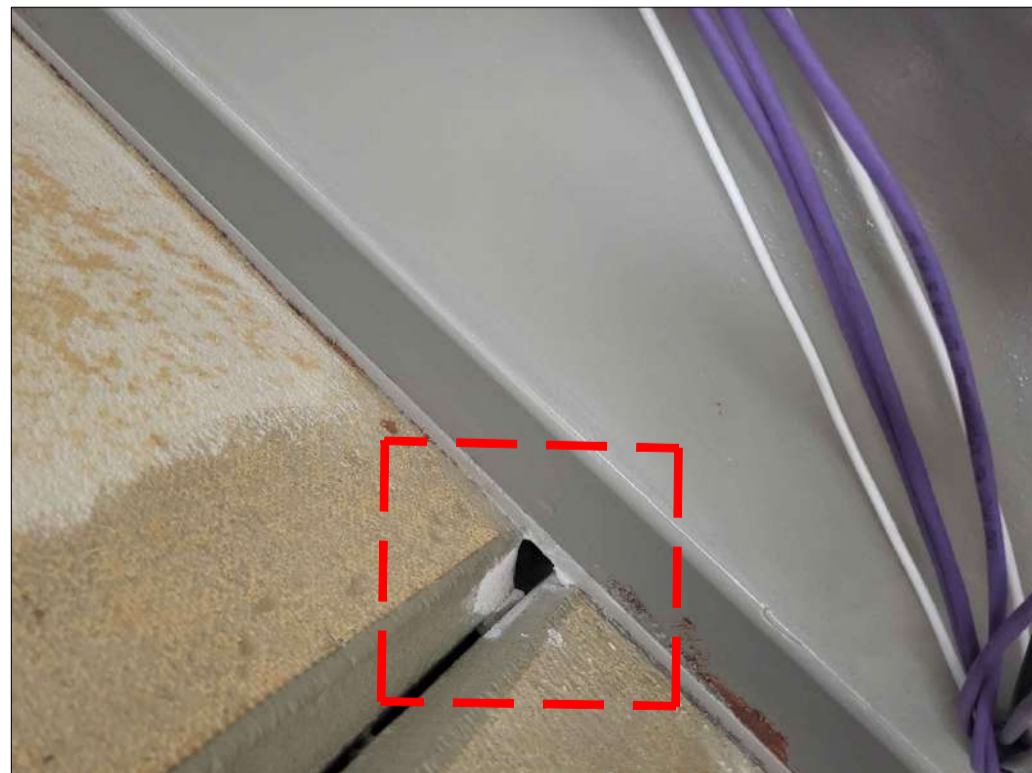
PHOTO 72 - PLANK No. 188 BROKEN EDGE AT END 1
