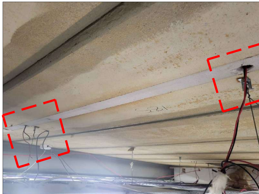
PHOTO 71 - PLANK No. 185 2No. SERVICE HOLES
