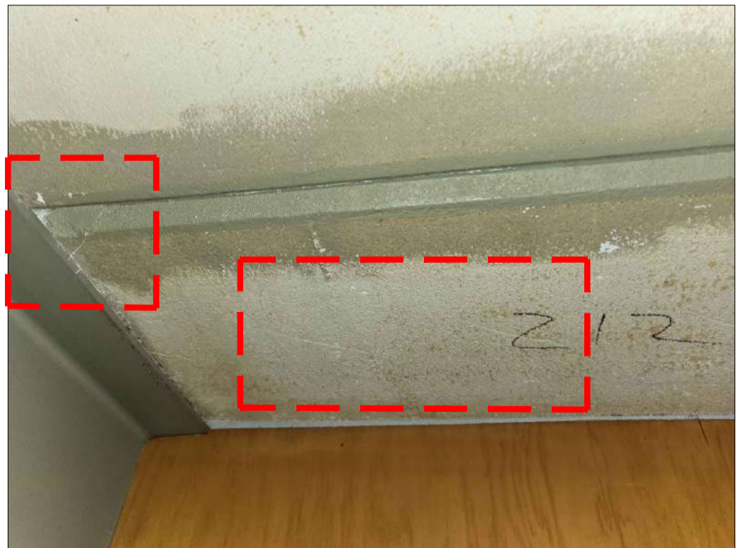
PHOTO 87 - PLANK No. 212 SCAR AT END 1 CRACK AT END 1
