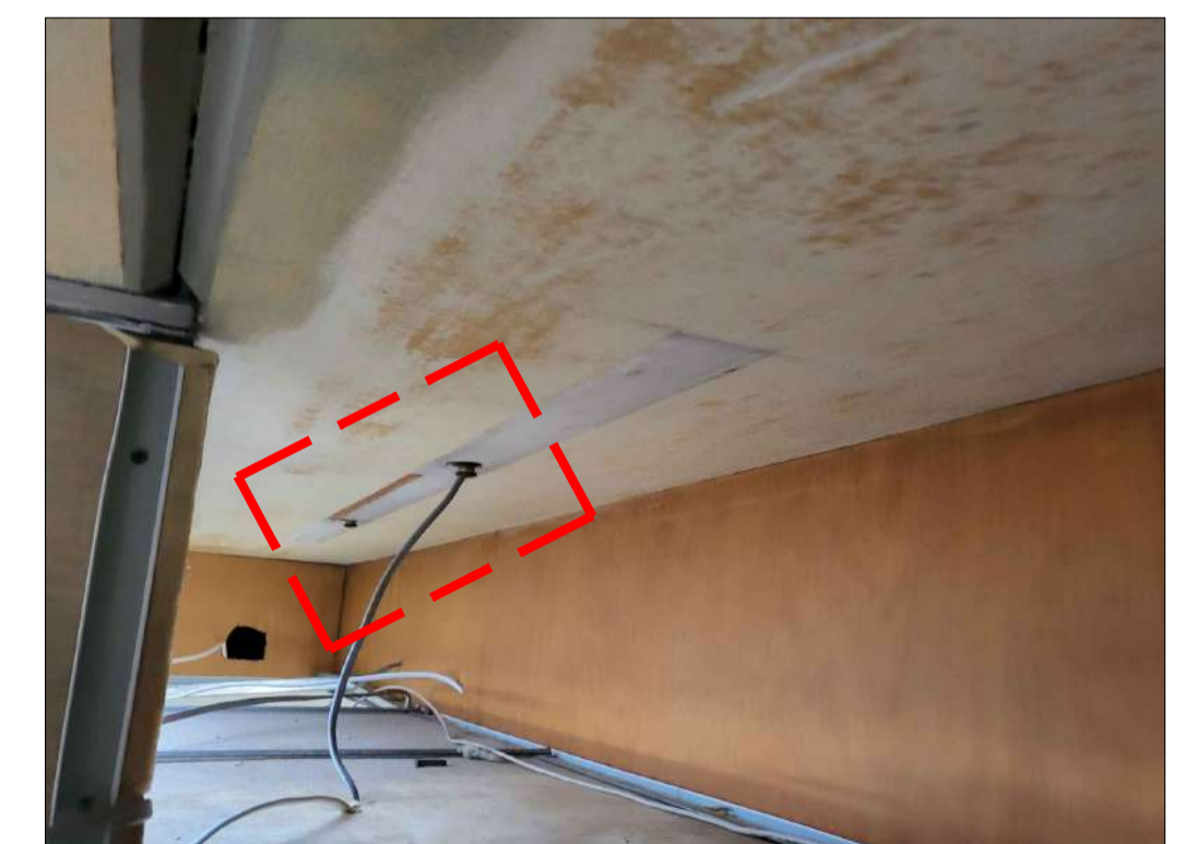
PHOTO 60 - PLANK No. 152 2No. SERVICE HOLES
