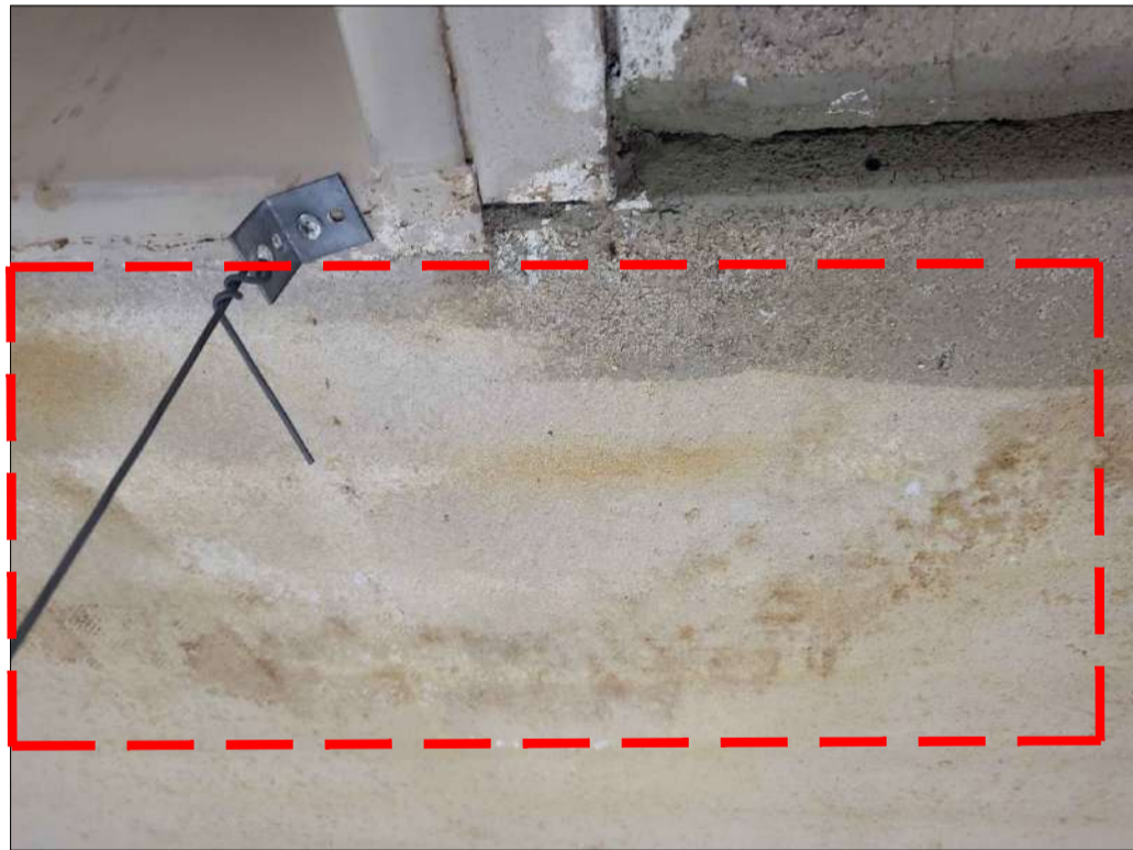
PHOTO 70 - PLANK No. 184 DELAMINATION WATER STAIN
