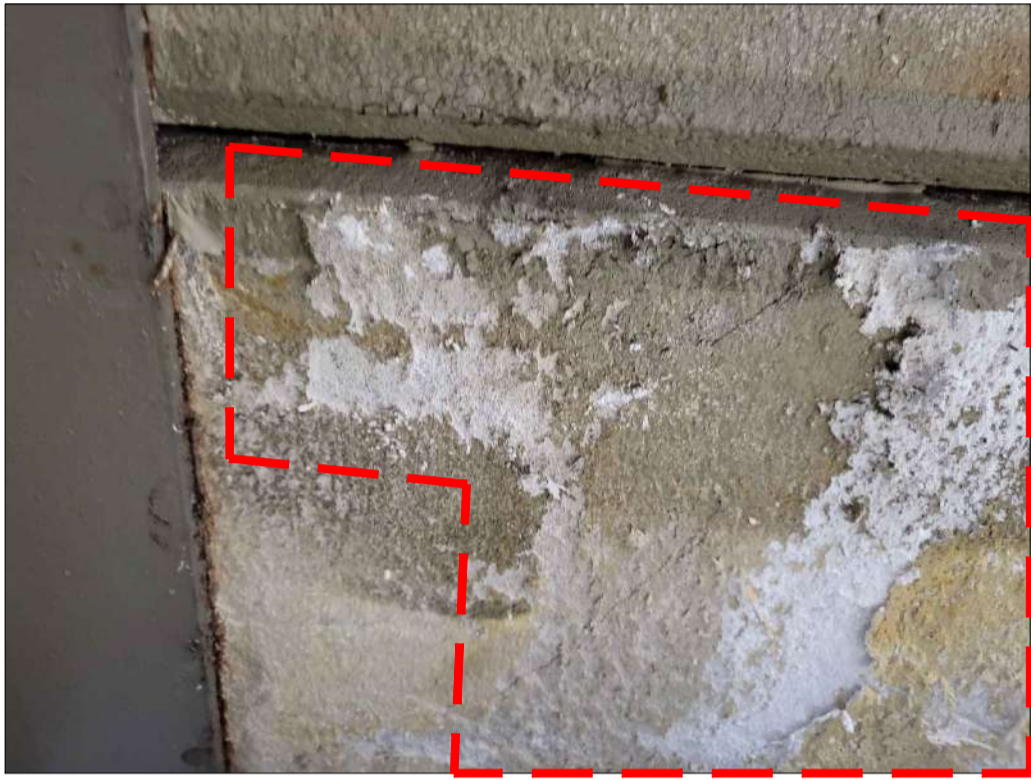
PHOTO 1 - PLANK No. 1 CRACKS & DELAMINATION/EFFLORESCENCE AT END 2
