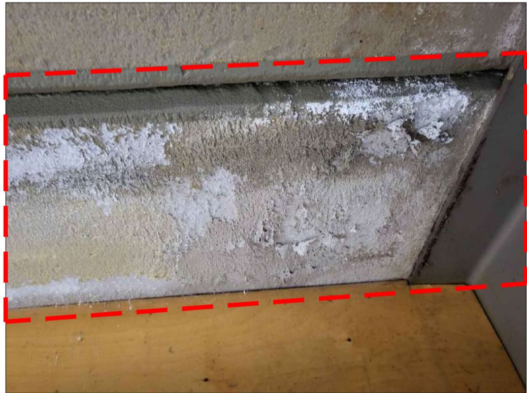
PHOTO 22 - PLANK No. 33 EFFLORESCENCE AT END 1
