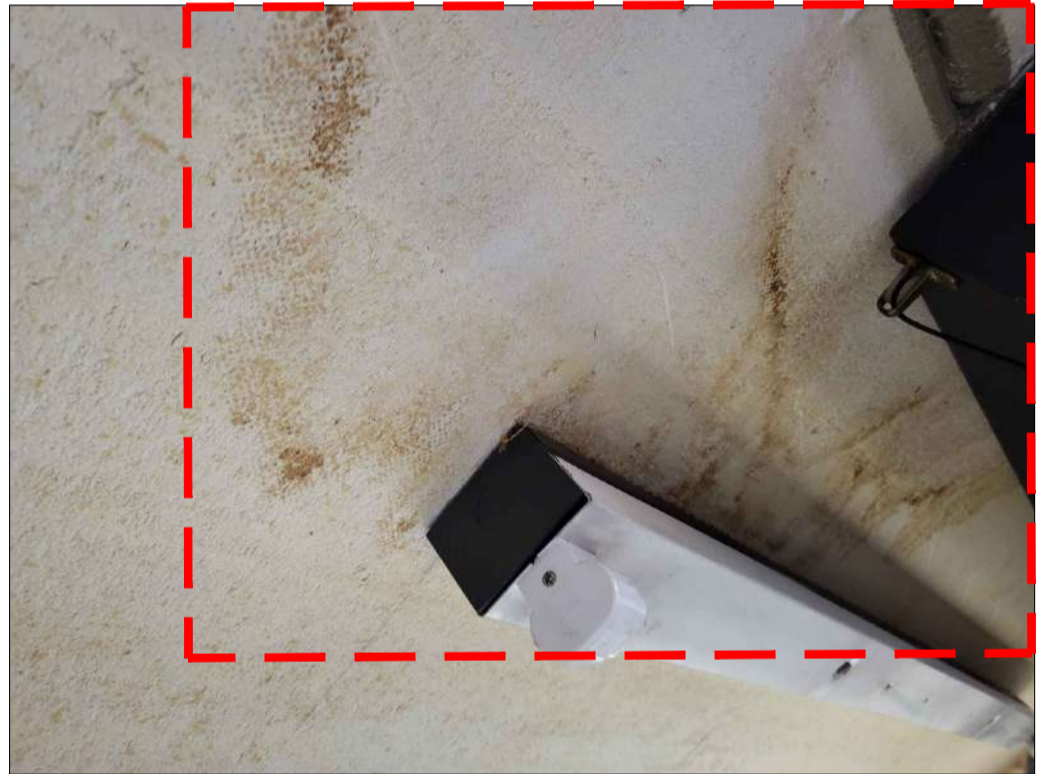
PHOTO 25 - PLANK No. 57 DAMP BY LIGHT
