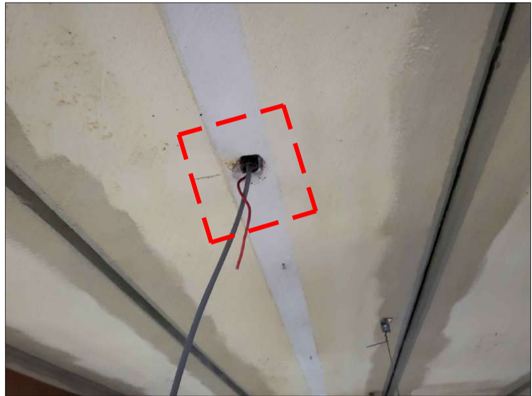
PHOTO 84 - PLANK No. 208 SERVICE HOLE
