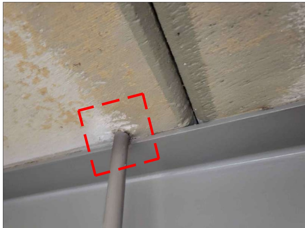
PHOTO 74 - PLANK No. 190 1No. HOLE AT BEARING
