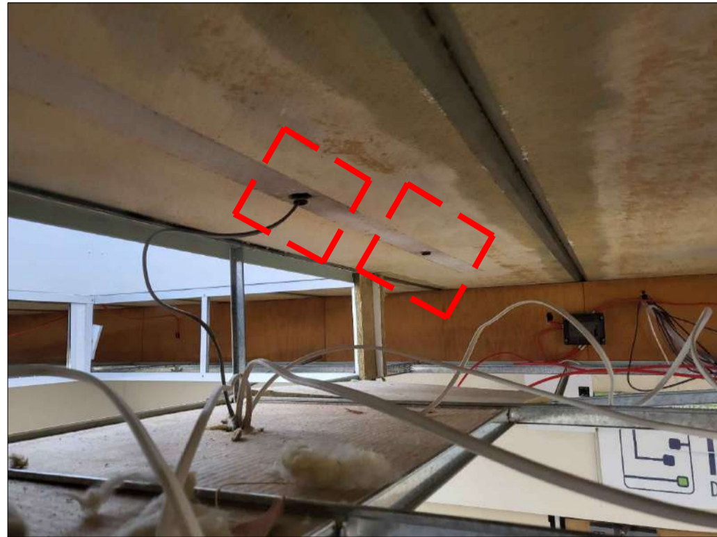
PHOTO 61 - PLANK No. 156 2No. SERVICE HOLES
