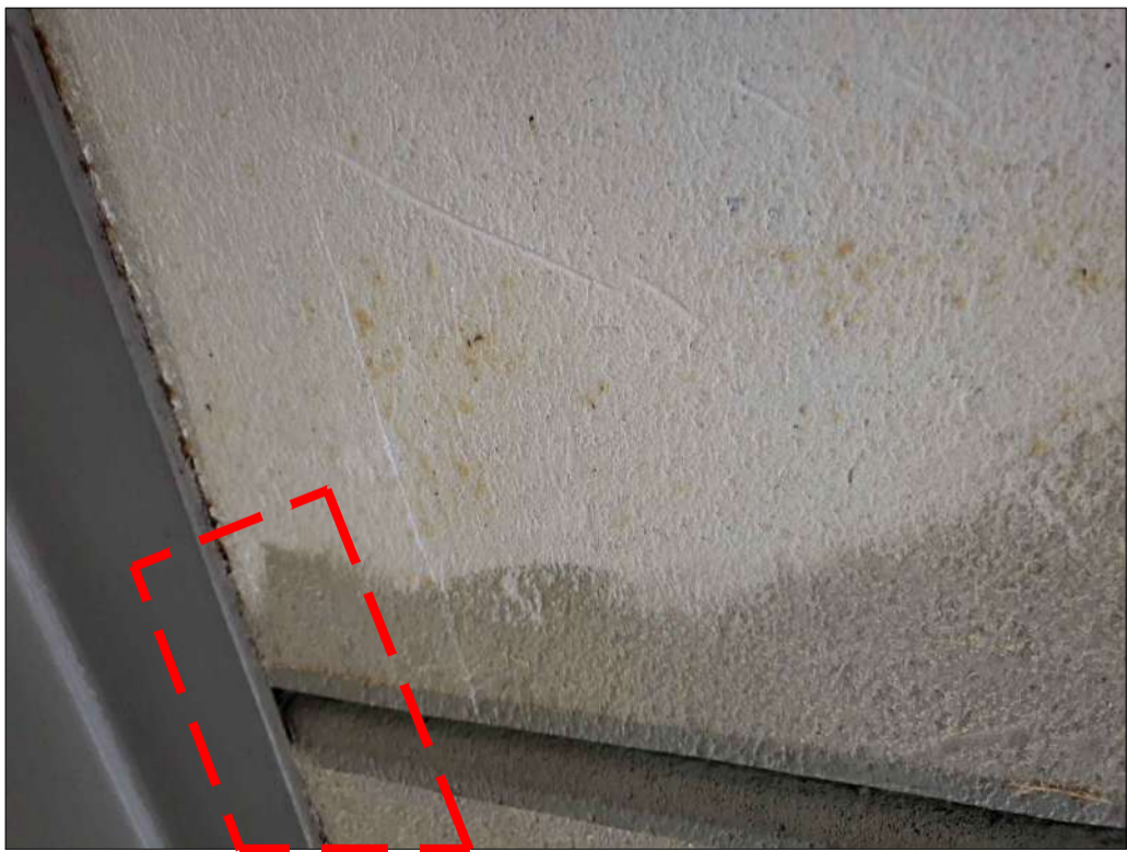
PHOTO 11 - PLANK No. 32 CRACK AT END 2
