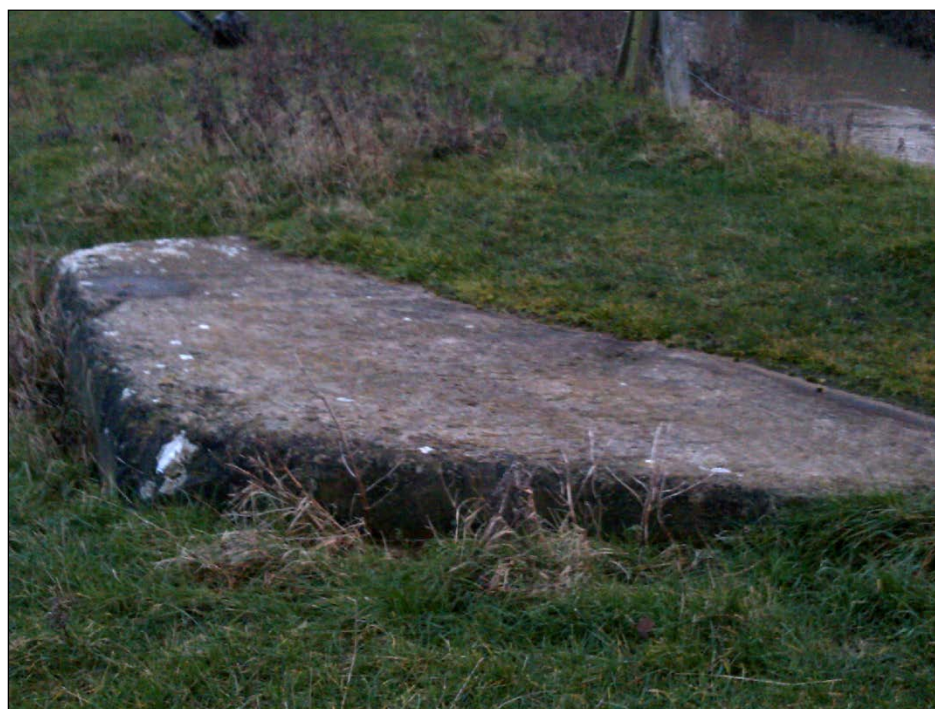
Figure 38. The sinking Longford pillbox type FW3/26 (NRHE: 1583785 ) in January 2014. © S. Crowther 2014.
