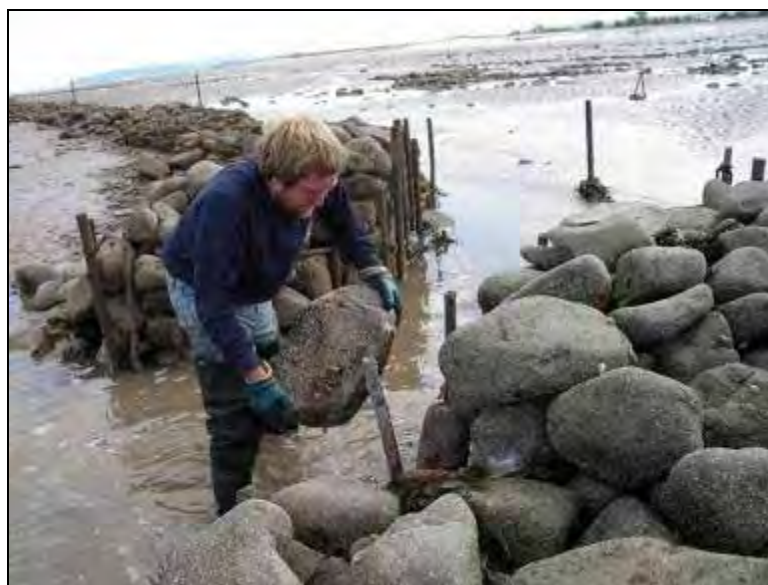
Figure 5.39. A stone weir at Minehead under much needed repair in 2007.
