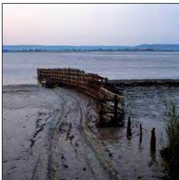
Figure 5.4. A putcher rank at Awre that is still in use, though steel has mostly replaced wood in basket construction.
