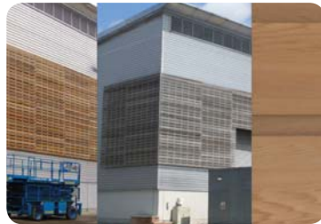
Fire treated Western Red Cedar boards spaced 50mm apart non-weathered and weathered.
