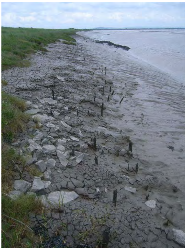
Plate 243: Stone and timber riverbank revetment on the western bank of the River Parrett north of Comwich, Som. ( Line No. 40021 ), similar to many within the Severn RCZAS area.
