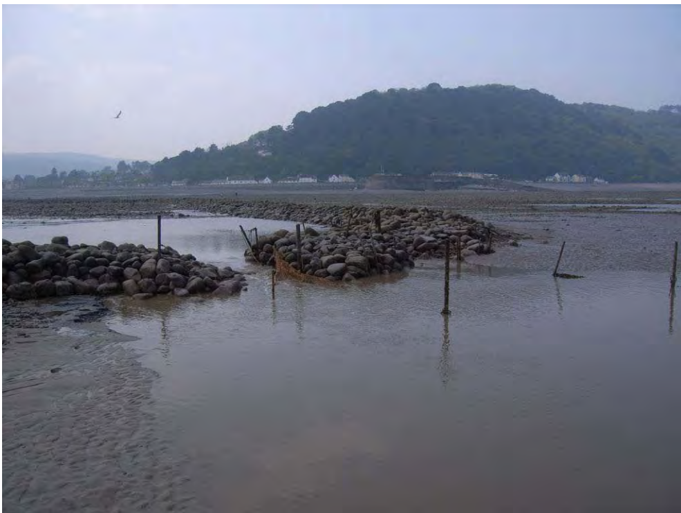
Plate 30: A well-defined gut or outflow channel on a stone fish weir at Minehead Bay, Som. (Line No. 10383). More metal scaffolding poles are present, and nylon netting.
