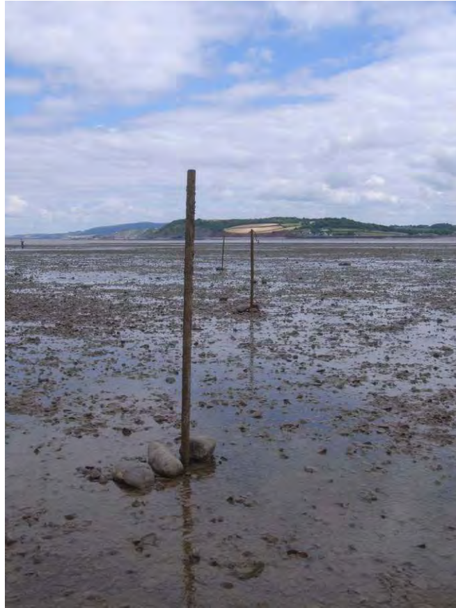
Plate 13: Stone rings or 'doughnuts' acting as net hang post supports for relatively recent metal poles at Blue Anchor Bay, Som. (not formally recorded).
