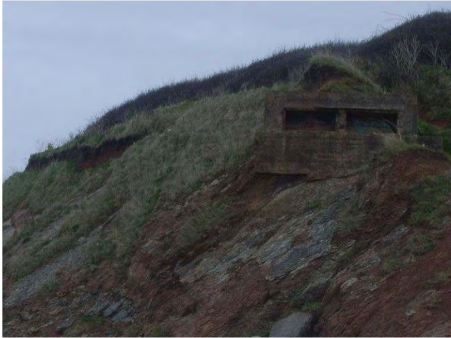
Plate 263: The concrete observation post on the eastern side of the harbour at Watchet, Som.; that will shortly fall off the soft eroding cliff face. It was not formally recorded.
