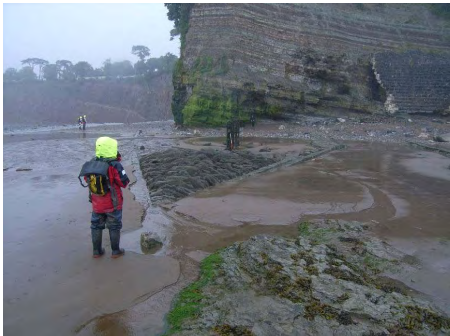
Plate 246: The stone and timber triangular breakwater or groyne at St Audrie's Bay, Som, originally designed to protect a grotto feature, partly visible at the right of the image.
