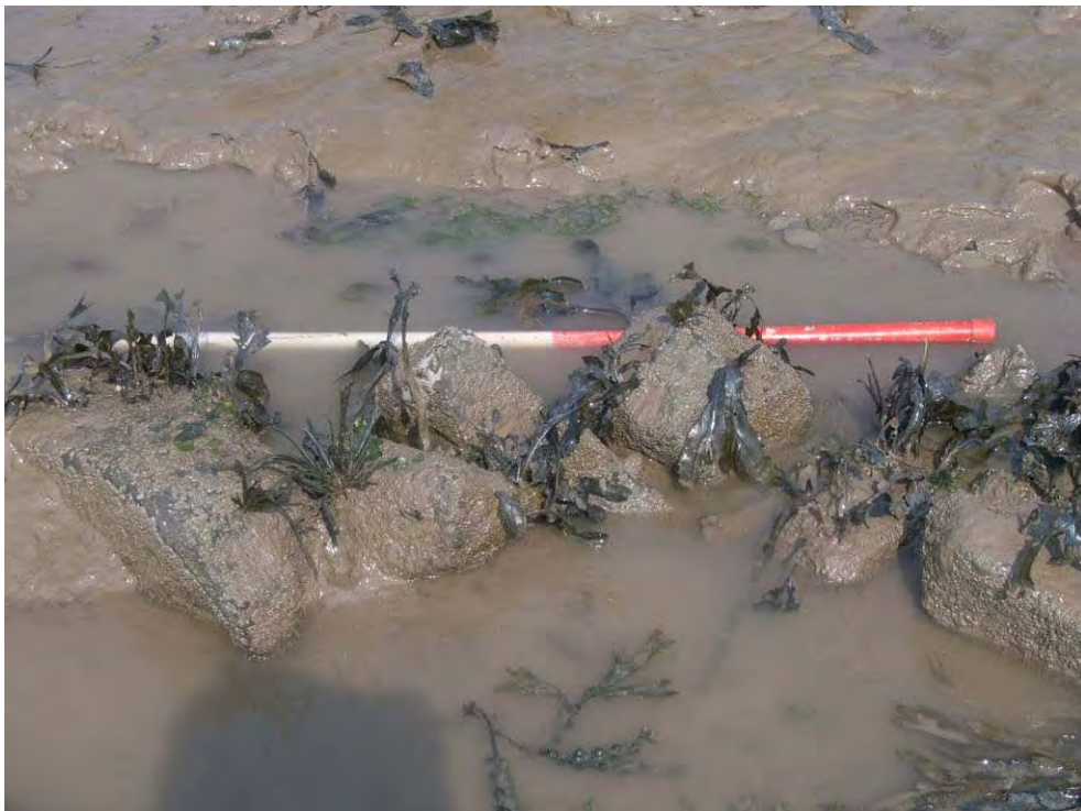
Plate 56: The stone filled leader arm of one of the small, rock-cut fish weirs at Stolford, Som.
