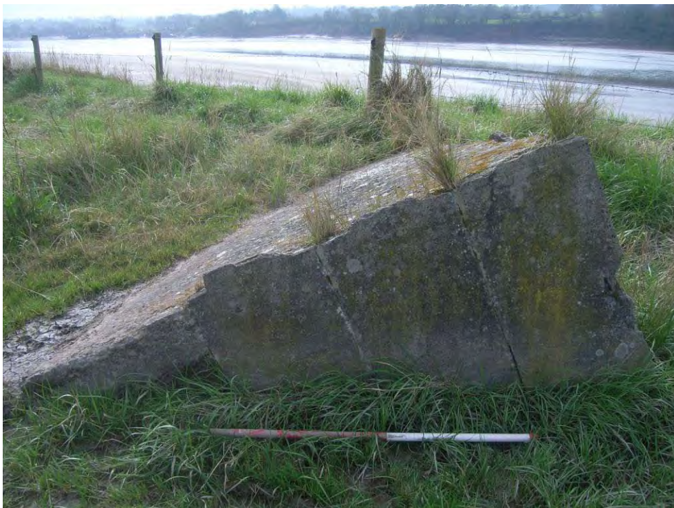
Plate 260: Another pillbox at Arlingham, Glos. ( Point No. 119 ), that has almost completely subsided into soft riverbank sediments south-west of Passage Farm.
