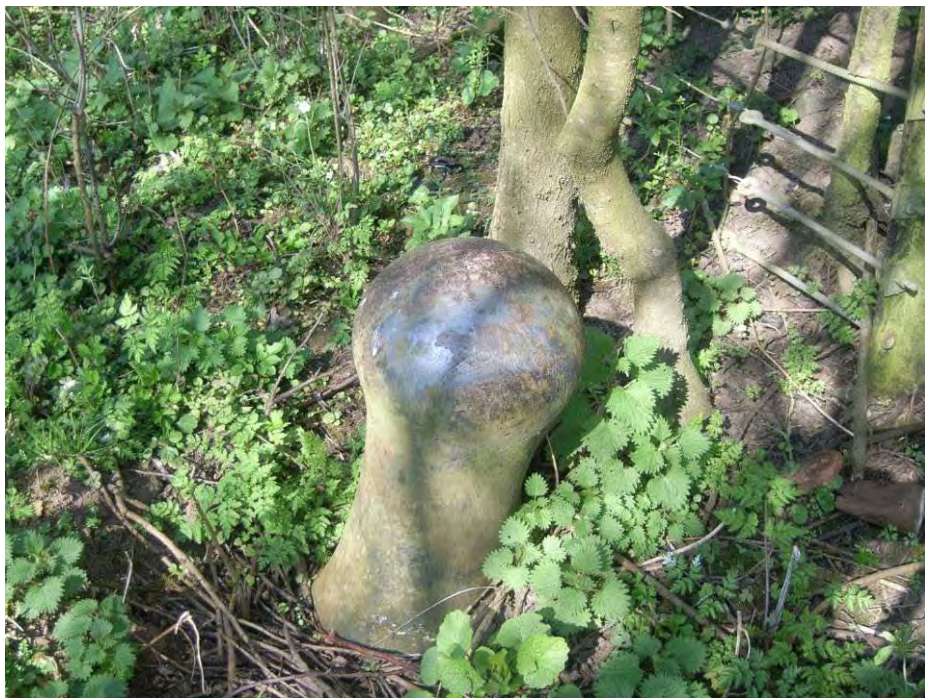
Plate 214: Purpose-made iron mooring post at Castle Meads, Alney Island near Gloucester. Originally used for canal boats to temporarily moor up, it is now overgrown in scrub.
