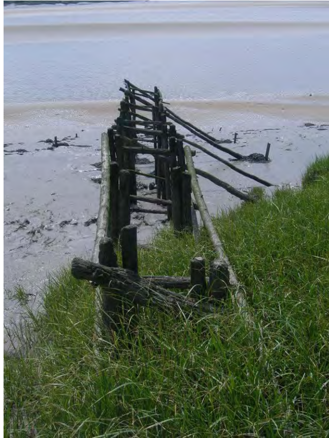
Plate 147: A 20 th century putcher rank at Gatcombe, Glos ( Line No. 10069 ), with surviving horizontal basket supports, as well as additional angled bracing timbers held by upright metal posts on the downstream side.
