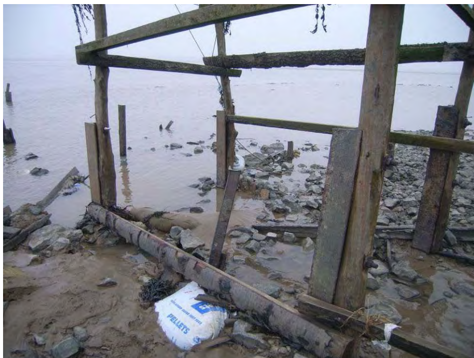
Plate 152: Another view of putcher rank Line No. 10350 north-east of Gatcombe, Glos, showing modern sawn timbers, steel pipes and angle irons all used in construction.
