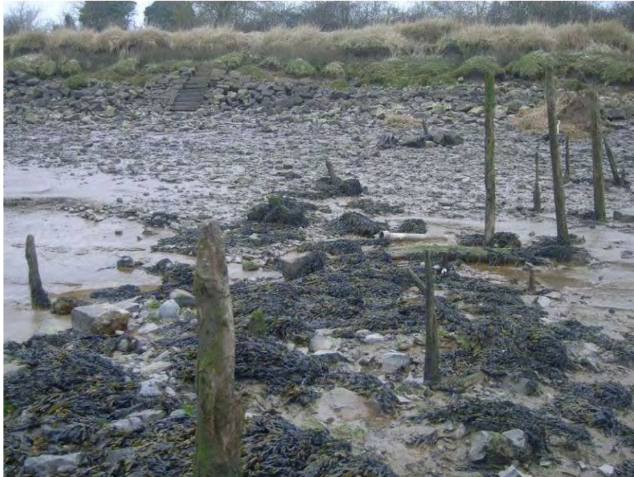
Plate 175: Putcher rank Line No. 10351 , south of Poulton Court, Awre parish, Glos. In the upper left, a flight of stone steps is visible, built into the flood defence wall.
