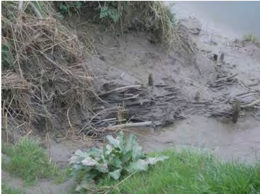
Plate 3: The side of one of the stake and wattling 'bays' identified in the riverbank near Elmore Back Farm, Gloucestershire.
